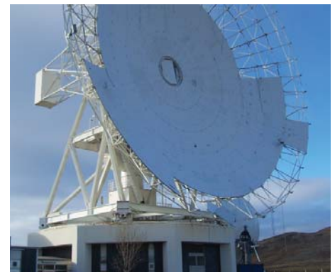
Communication network management centers
